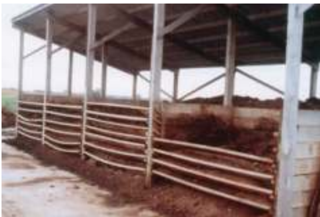
Figure 5. This simple four-bin swine mortality composting unit includes space for dry storage of cover material behind the bins. (Photo by Palmer Holden, Iowa State University.)
